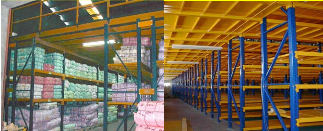
RACK SUPPORTED MEZZANINE
